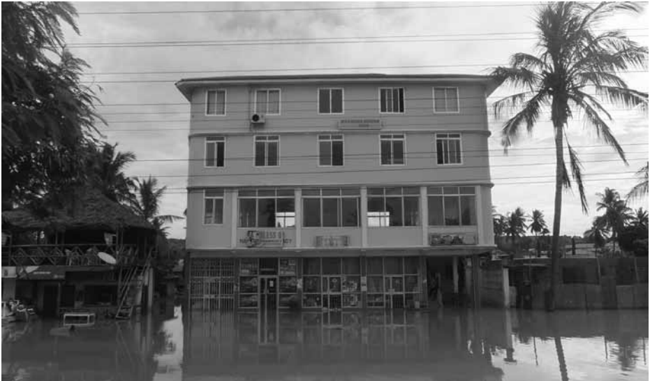
Flooded buildings on Bagamoyo Road, Dar es Salaam
