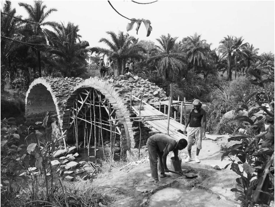
Stone arch construction in Kigoma region - newcivilengineer.com
